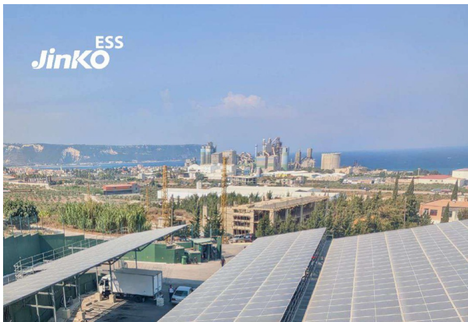
Fig. 11: Carport PV plant at the facility, with the Chekka coastline in the background
